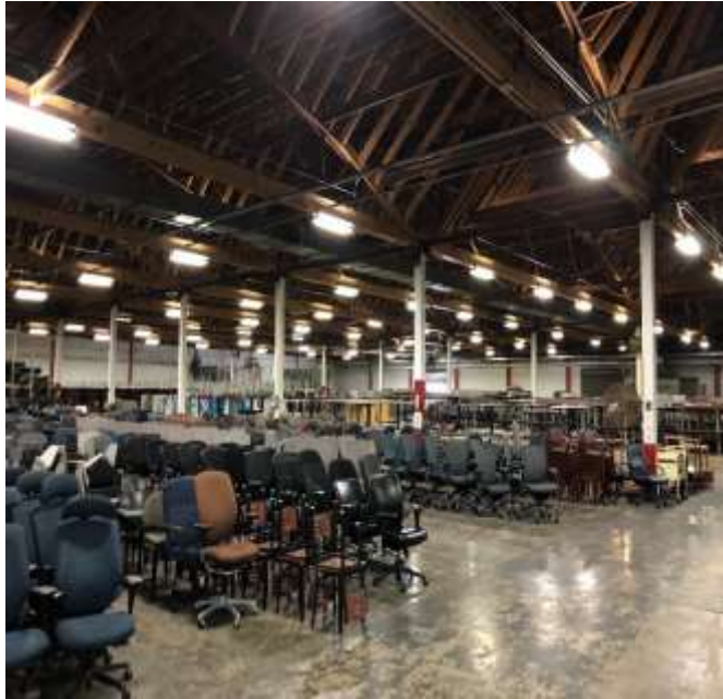
Image 1 - Floor storage for larger items
