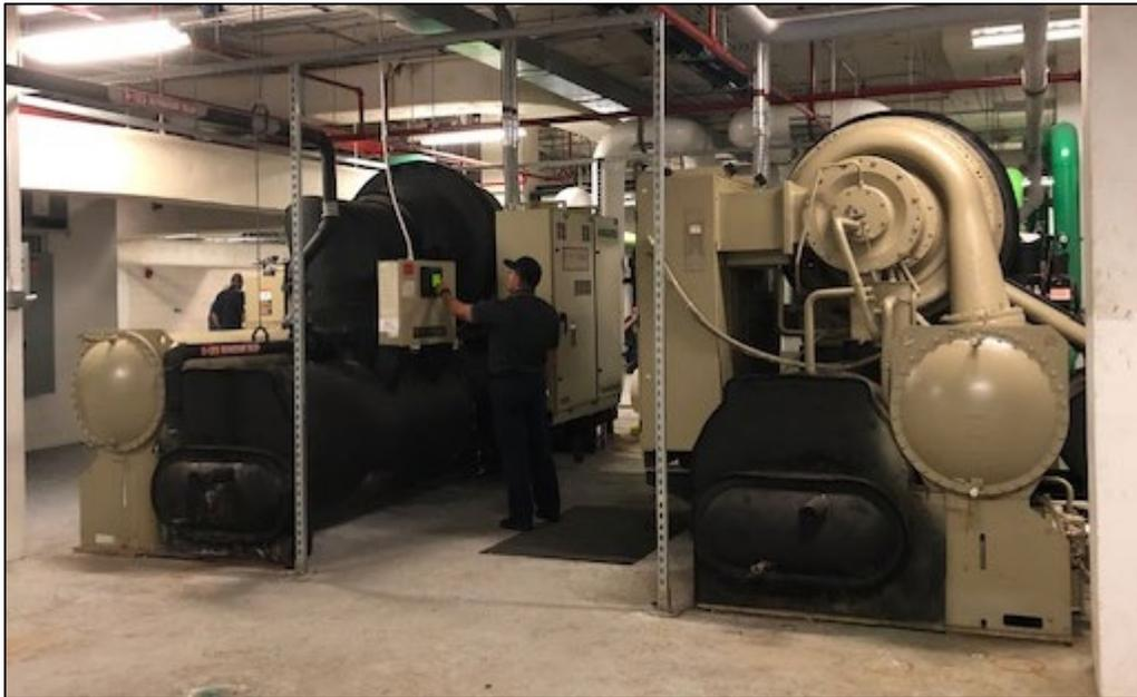
Chillers cool buildings by removing heat from a liquid coolant to cool and dehumidify the air. A breakdown in a chiller may lead to rising temperatures and humidity within the building and possible building closures.
