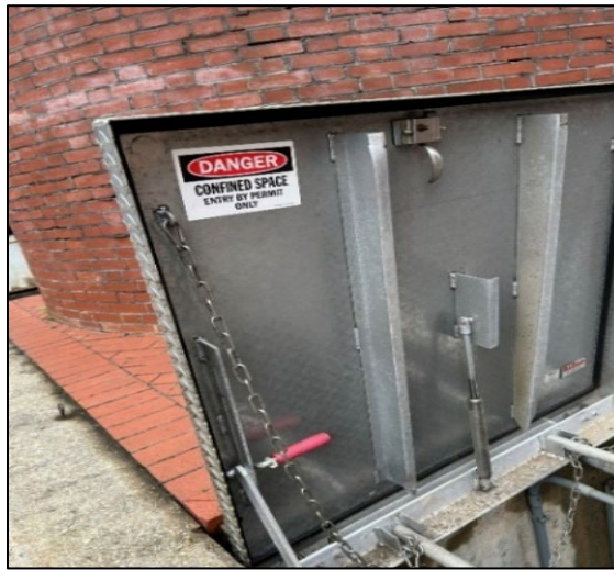
Figure 3. Cooling Tower Entry Gate at the Sidney R. Yates Federal Building with Permit Space Label Added 11
