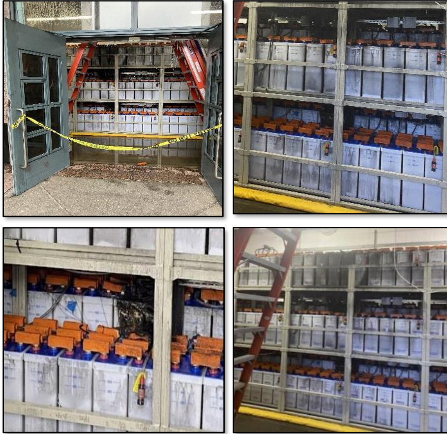
Figure 10. Post-Fire Photos of the Anderson Building Battery System 23
