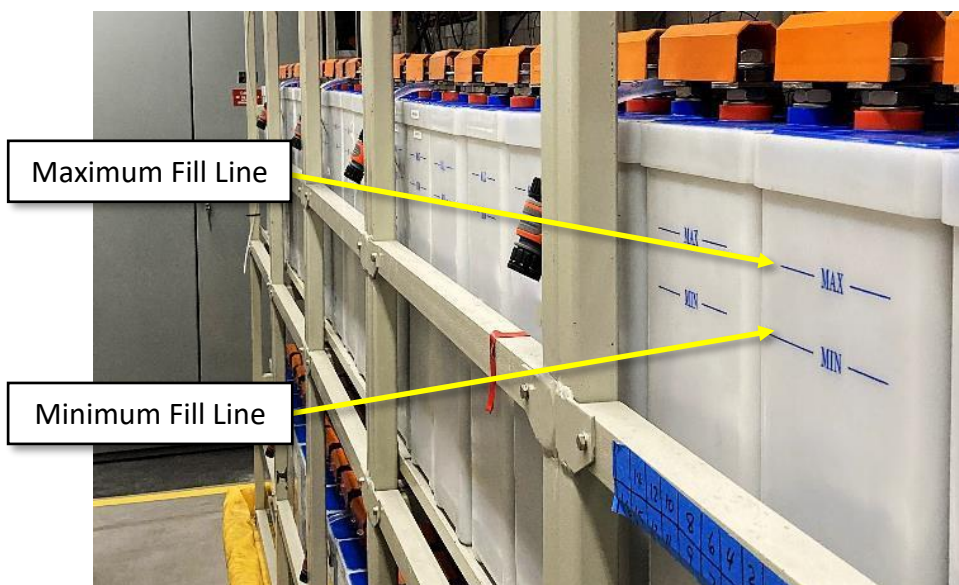
Figure 7. Nickel-Iron Battery Cells Showing Maximum and Minimum Fill Lines at the Reagan Building 10
