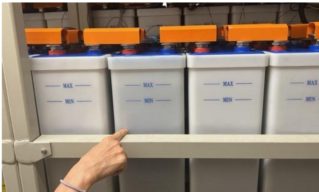
Figure 8. Defective Nickel-Iron Battery Casings at the Reagan Building 14
