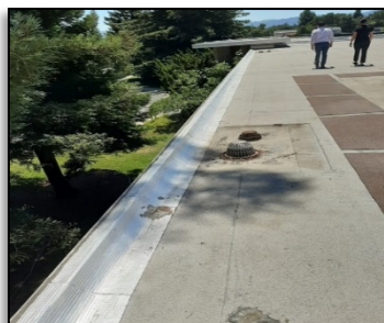
Figure 2 – Photograph at USGS campus showing no fall protection
