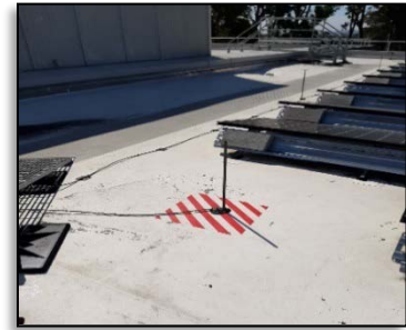
Figure 1 – LPS rods at Leo J. Ryan Federal Records Center
