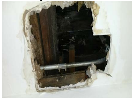
Figure 6: Open ceiling area in the third floor training room.
