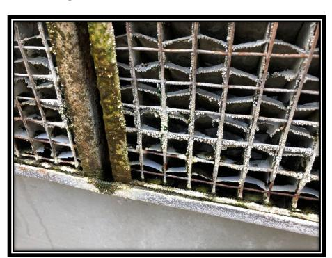
Figure 4 – Biological Growth and Scaling on the Cooling Tower at the Sam Nunn Atlanta Federal Center<sup>9</sup>
