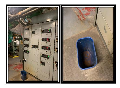
The O&M contractor marked the work order in NCMMS as being completed on November 14, 2022. However, as shown in *Figure 3*, the leak was not fixed; therefore, the O&M contractor did not complete the work.
