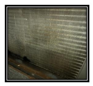
NCMMS indicated that preventive maintenance on the AHU was completed in April 2023. Despite the condition of the AHU coils during our visit on May 18, 2023, the contractor still marked the work order as complete in NCMMS. However, the contractor did not complete the preventive maintenance properly, like the COR experienced in June 2022.
